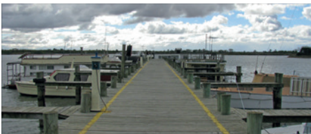
Berthing at a jetty
